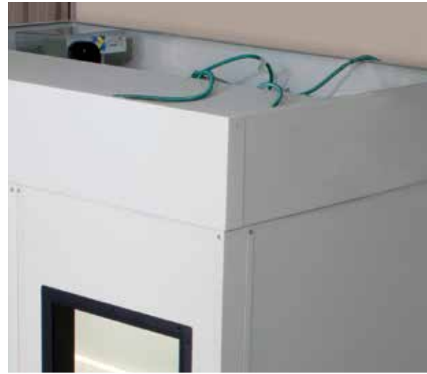
Ceiling Soffit Provides a Cleaner Line of Sight
